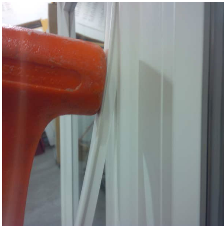
Figure 5: Attaching capping to window exterior using mallet
