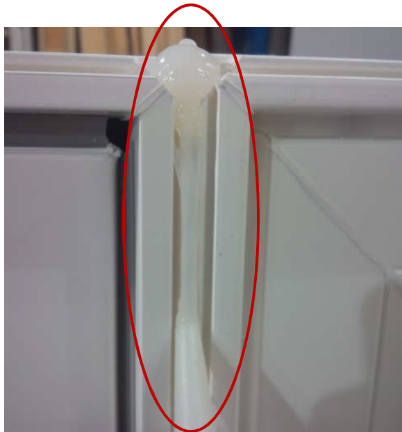
Figure 2: Silicone sealant applied along exterior joint, where Windows come together.
