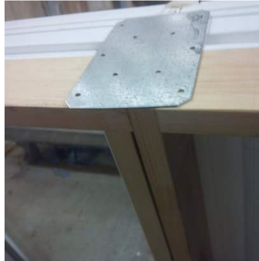
Figure 8: Positioning of mending plate on attachment point
