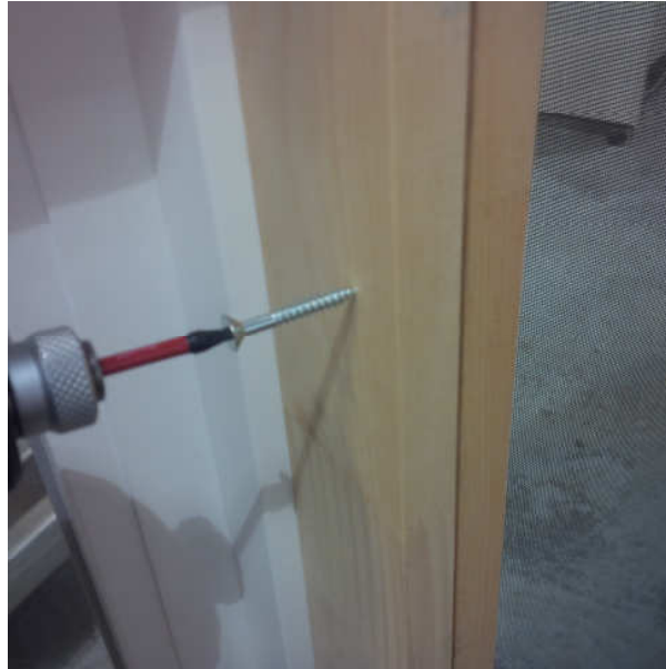
Figure 6: Fasten interior extensions using #8 x 1-1/4" screws
