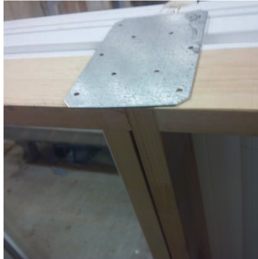
Figure 8: Positioning of mending plate on attachment point
