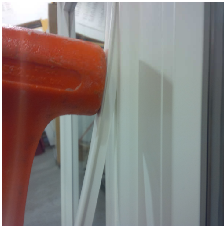
Figure 5: Attaching capping to window exterior using mallet
