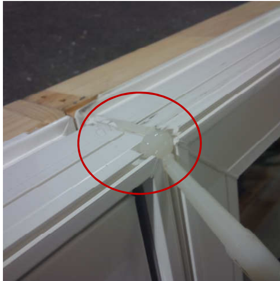
Figure 1: Silicone sealant applied across exterior edge of product, and corner cleaned area.
