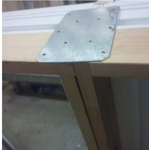
Figure 8: Positioning of mending plate on attachment point
