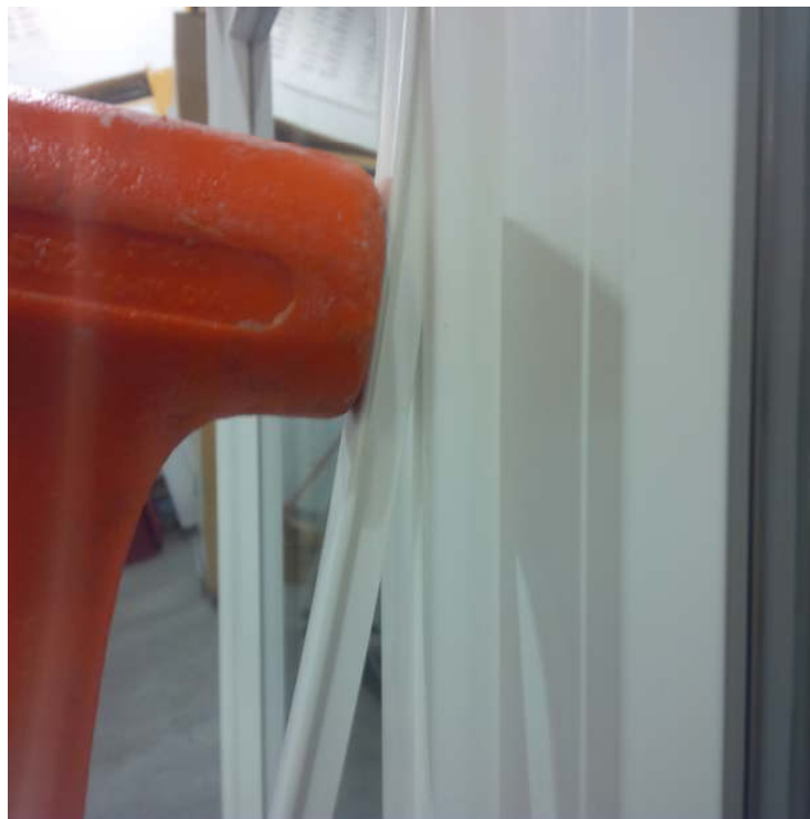
Figure 5: Attaching capping to window exterior using mallet
